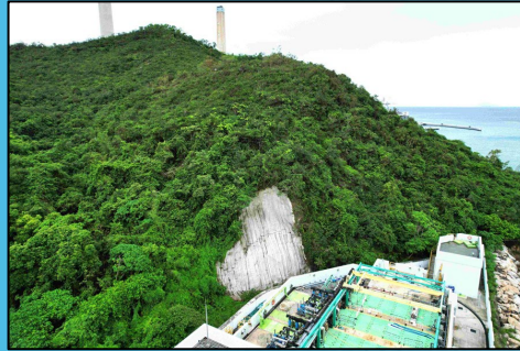
Slope Protection at Lamma Island August 2024 (GE/2022/05)
