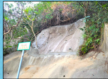
Slope Protection, Highways Term Contract, August 2025 (06/HY/2017)
