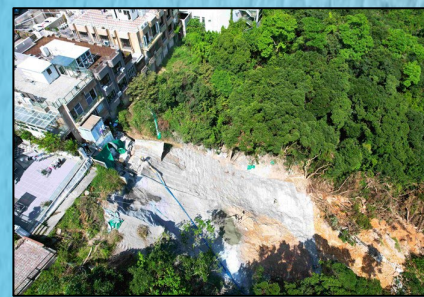
Temporary Slope Protection in Hilltop Villa, September 2023
