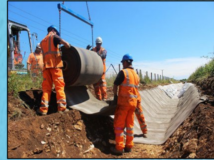
Laying of Concrete Canvas
