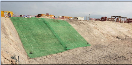
Erosion mat secured by Platipus anchor 3 rd runway, Hong Kong
