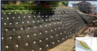
Slop stabilization and erosion mat anchor
