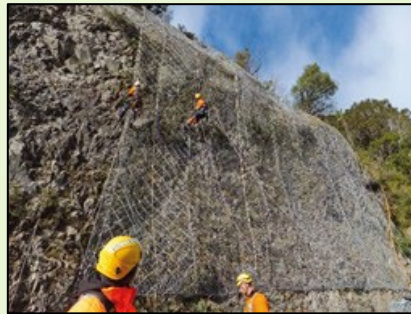
Rock slope stabilization
