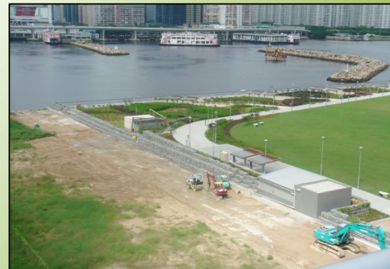
Embankment Protection June 2014
