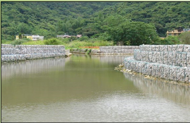
Drainage improvement, May 2010
