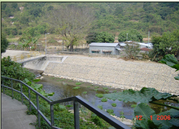
Improvement to Lam Tsuen River, January 2006
