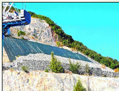
Gabion Buttress December 2023
