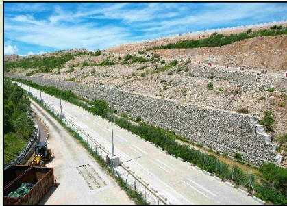
Soil Retainment Butress June 2025
