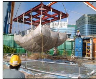
Handling filled Concrete Mattress
