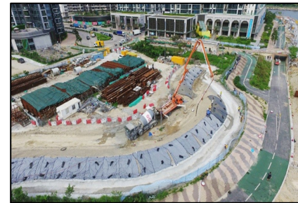
Embankment protection at Tseung Kwan O, April 2019
