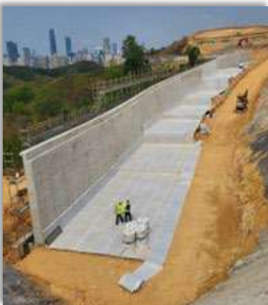
Retaining wall drainage at Police Facilities in Kong Nga Po March 2021 (ND/2018/01)
