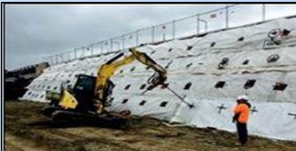
Temporary embankment stabilization
