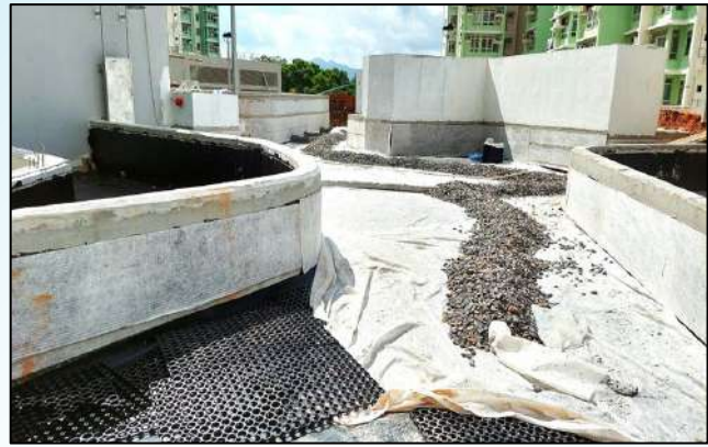
Drainage Layer, PHD at Tai Po Area 9, August 2024 (HKHA20190169)
