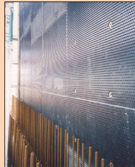
Studliner on formwork
