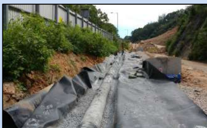
Hiram's Highway Improvement November 2018 (HY/2014/16)
