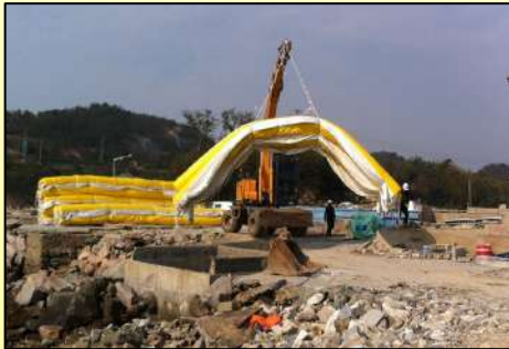
Handling of the silt curtain
