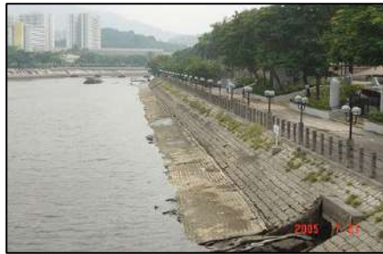
Shing Mun River scouring protection, July 2005
