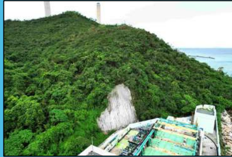
Slope Protection at Lamma Island August 2024 (GE/2022/05)
