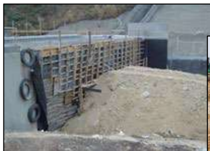
Mechanical Stabilized Earth Wall (MSEW) (2007)
