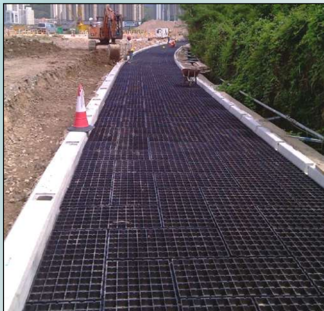
Installation of Geoblock 5150 at Tseung Kwan O Stage 1 Landfill Site
