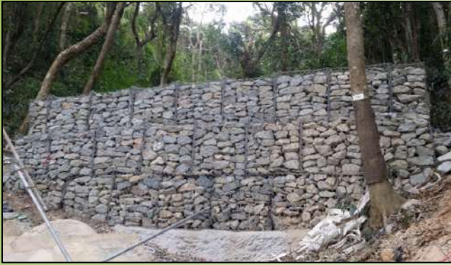
LPM, Luard Road, November 2015
