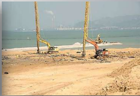
Hong Kong-Zhuhai-Macau bridge – HK Boundary Crossing Facilities. Feb 2014 (HY/2010/02)
