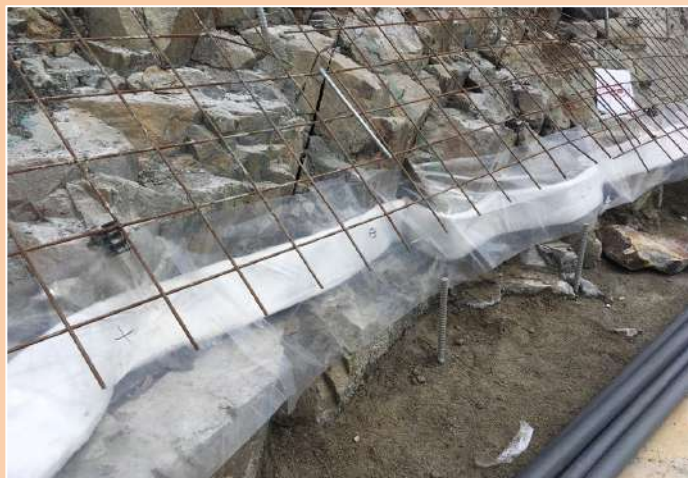
Relief drain at Anderson Road Quarry Development
