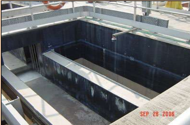
Outlying Islands Sewerage, Siu Ho Wan DC/99/10, September 2006
