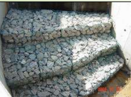
Drainage Improvement November 2008
