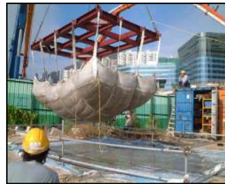
Handling filled Concrete Mattress
