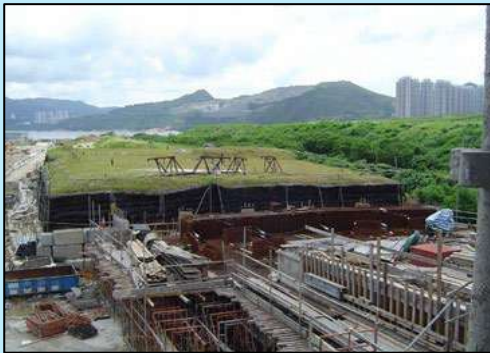
Surcharge Bund at Residential Development at Wo Shang Wai, Yuen Long, 2012
