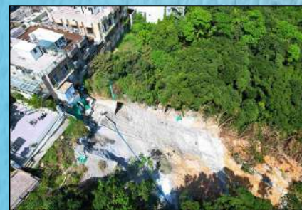
Temporary Slope Protection in Hilltop Villa, September 2023
