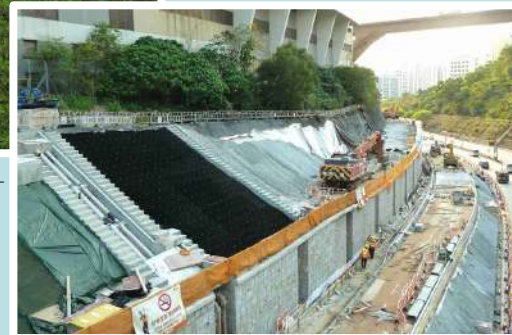
Soil Retainment for Landscaping on slope – Anderson Road Quarry Site – Road Improvement Works. March 2025 (NE/2017/03)
