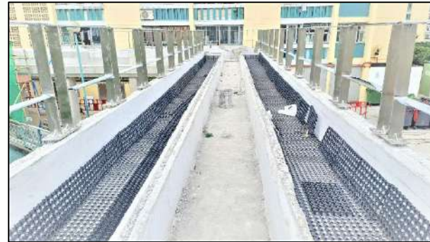
Planter Drainage, Ching Hong Road
