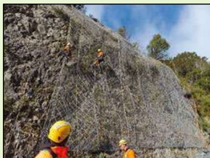
Rock slope stabilization
