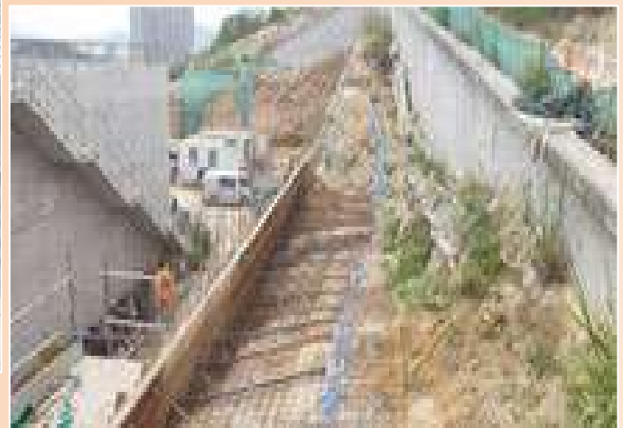
Relief drain at Anderson Road Quarry Development
