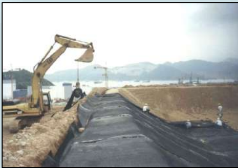
SENT Landfill, December 2001
