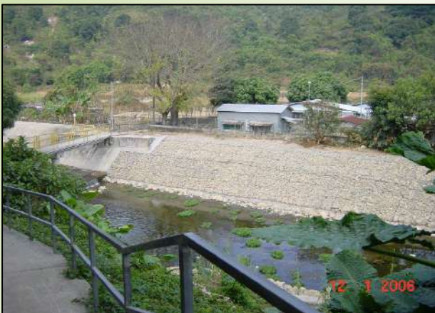
Improvement to Lam Tsuen River, January 2006
