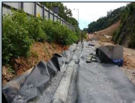
Hiram's Highway November 2018
