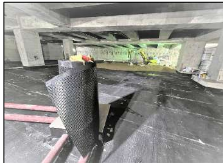
Basement slab drainage at No. 53 – 55A Kwun Tong Road Development August 2022
