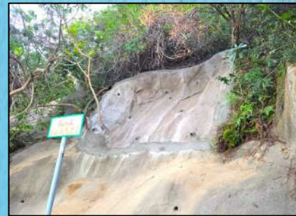
Slope Protection, Highways Term Contract, August 2025 (06/HY/2017)
