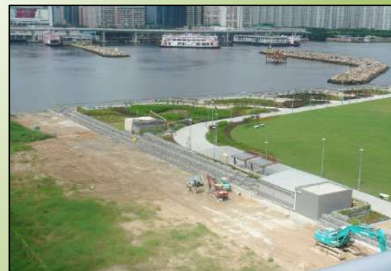
Embankment Protection June 2014
