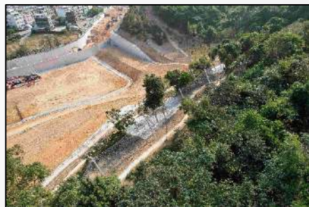
Site Formation at Cheung Muk Tau CV/2023/09, February 2026
