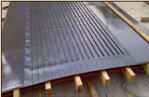
T-Keyed liner on timber formwork
