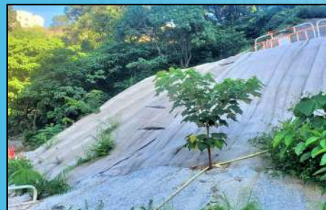
Slope Protection in Pik Wan Road, April 2021 (CV/2019/03)
