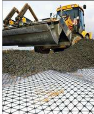
Composite Geogrid with Geotextile Reinforcement and Separation
