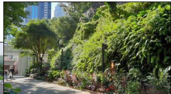
Hong Kong Park Reinforced Fill Slope (2021)
