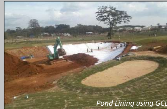
Installation of GCL
