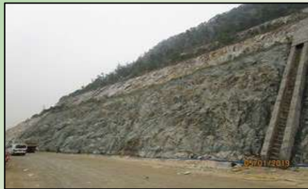
Erosion Control at Anderson Road Quarry, March 2019
