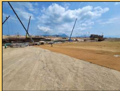
Third Runway Concourse May 2022 (C3405)
