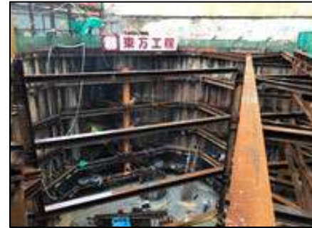
Basement Vertical Drainage Tsuen Wan, August 2019
