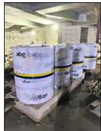
Packed material on site
