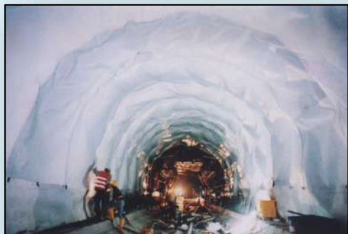
Lam Tin Tunnel February 2001
