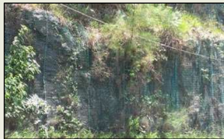
Erosion Control at Tolo Highway August 2012
