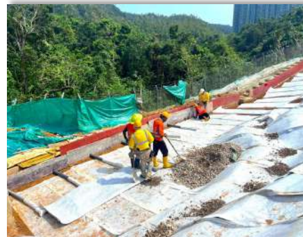
Fill Slope Drainage at TKO - Yau Yue Wan, October 2023 (CV/2021/04)
