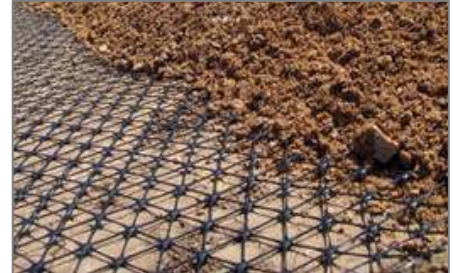
Tri-Axial Geogrid Ground Stabilization in Weak Subgrade
