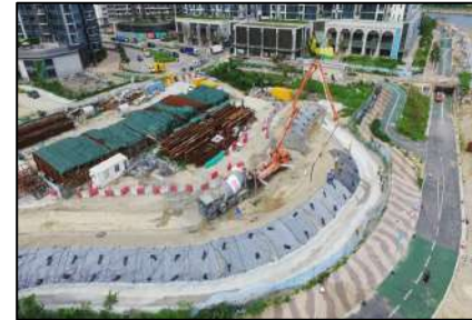
Embankment protection at Tseung Kwan O, April 2019
