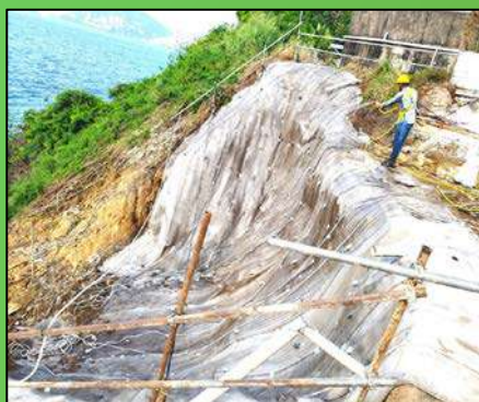
Lamma Island Pak Kok Village - eroded surface being covered instantly
