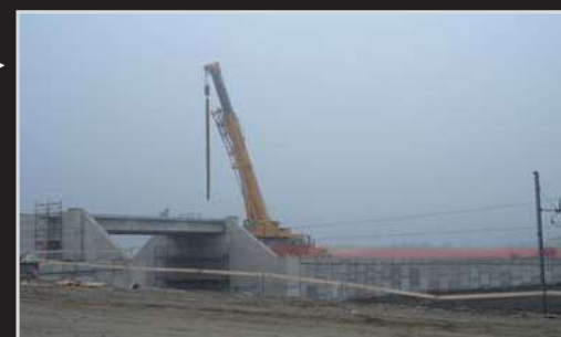
Railway overpass Fidenza (Italy) -Italferr SpA
