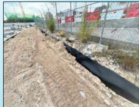
Root Barrier, Anderson Road Quarry, October 2022 (NE/2016/01)
