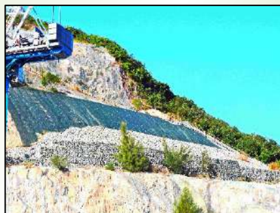
Gabion Buttress December 2023
