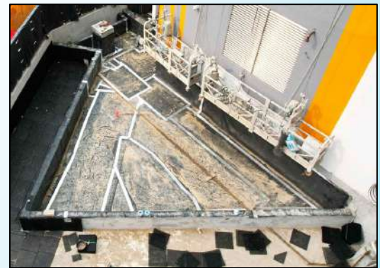
Planter Waterproofing, PHD at Wang Chiu Road, January 2026 (HKHA20210526)
