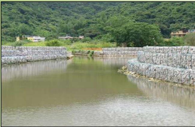
Drainage improvement, May 2010
