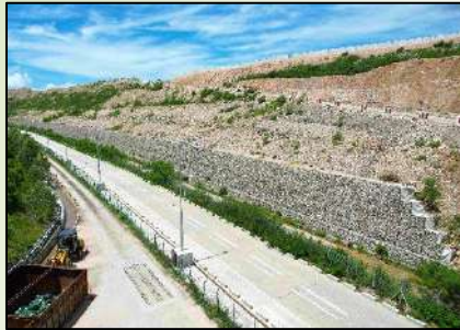
Soil Retainment Buttress June 2025
