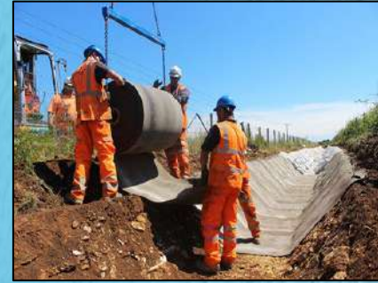
Laying of Concrete Canvas
