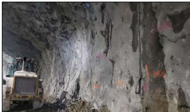
Tunnel Drainage, Shatin Sewage Treatment Works to Caverns, November 2020 (DC/2018/05)
