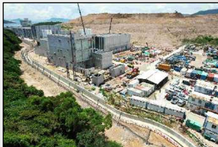
Desalination Plant at TKO 13/WSD/17, August 2023
