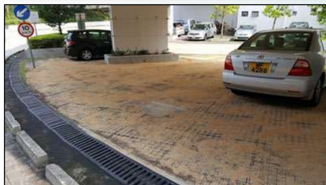
Landscape Paving for Fire Access at Shatin Transfer Station, May 2017 (EP/SP/76/14)
