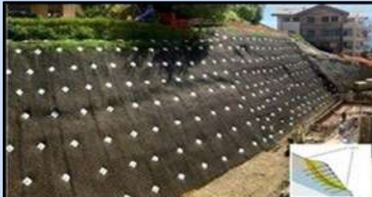
Slope stabilization and erosion mat anchor
