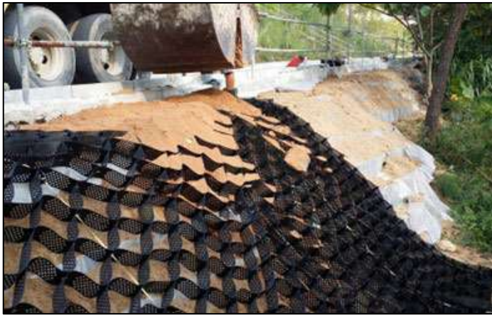
Geocell stabilizes the soil, which allows vegetation to thrive. (DC/2007/12)
