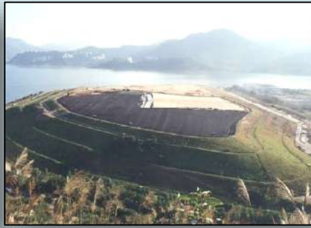
Shuen Wan landfill, December 2001
