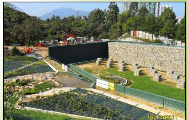
LPM, Cheung Tung Road, March 2013
