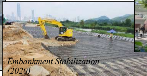
Composite Geogrid with Geotextile Reinforcement and Separation
