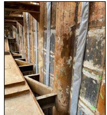
Basement Drainage Network Kwun Tong, March 2021
