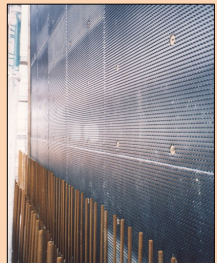
Studliner on formwork
