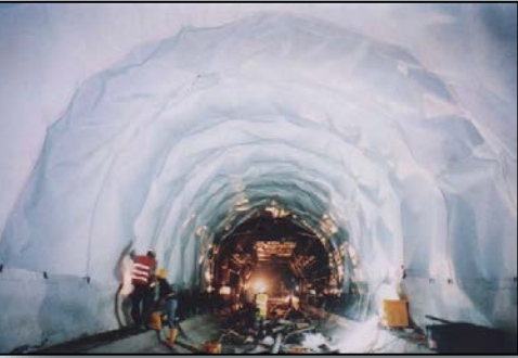
Lam Tin tunnel, February 2001
