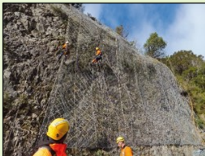
Rock slope stabilization
