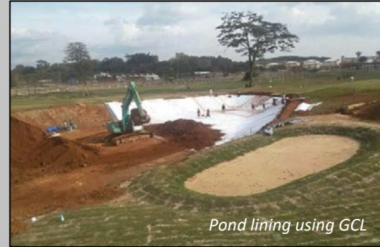
Installation of GCL
