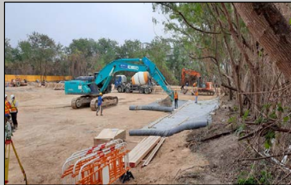
Wetland waterproofing January 2022 (YL/2020/02)
