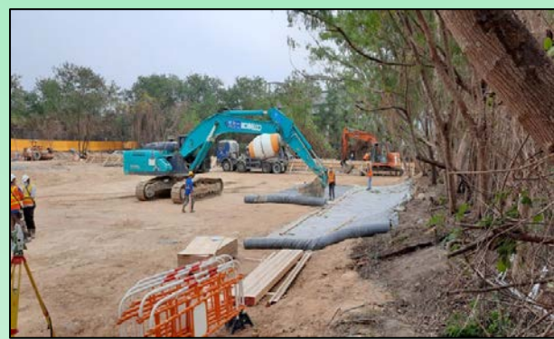
Wetland waterproofing January 2022 (YL/2020/02)
