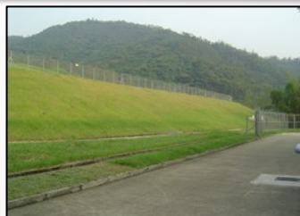
Erosion control at Tseung Kwan O Landfill Restoration, 2007
