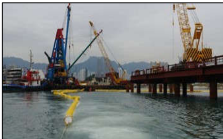
Silt Curtain trained to position, HY/2014/07
