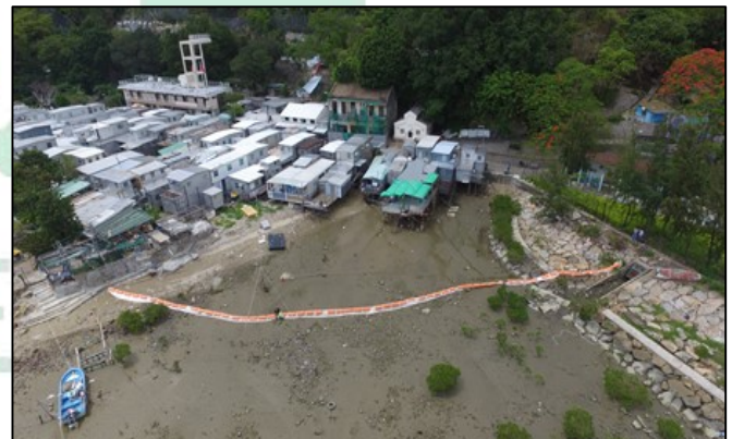
Completion at low tide
