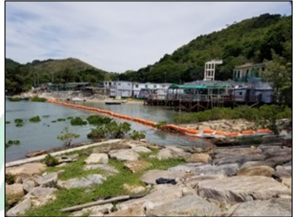
Fencing off the Stilt house
