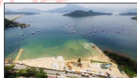
Fabrication from Bontec SG110/110 geotextile (CV/2012/05)
