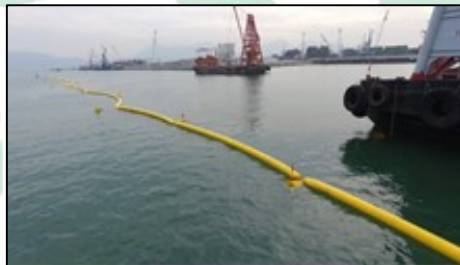
Heavy duty Korean tube type that stretches to 10 m depth (HY/2012/08)
