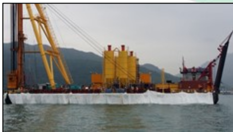
A high strength reinforced woven geotextile that can be attached to barge, retractable by winch (C3204)
