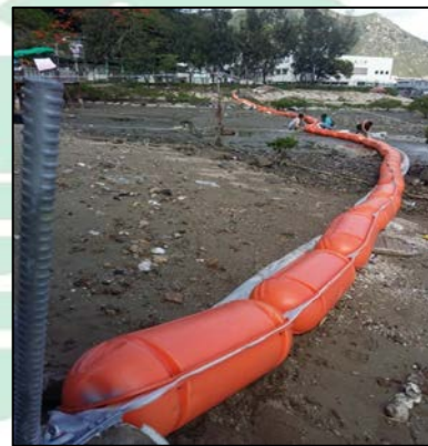
Installation of the refuse boom
