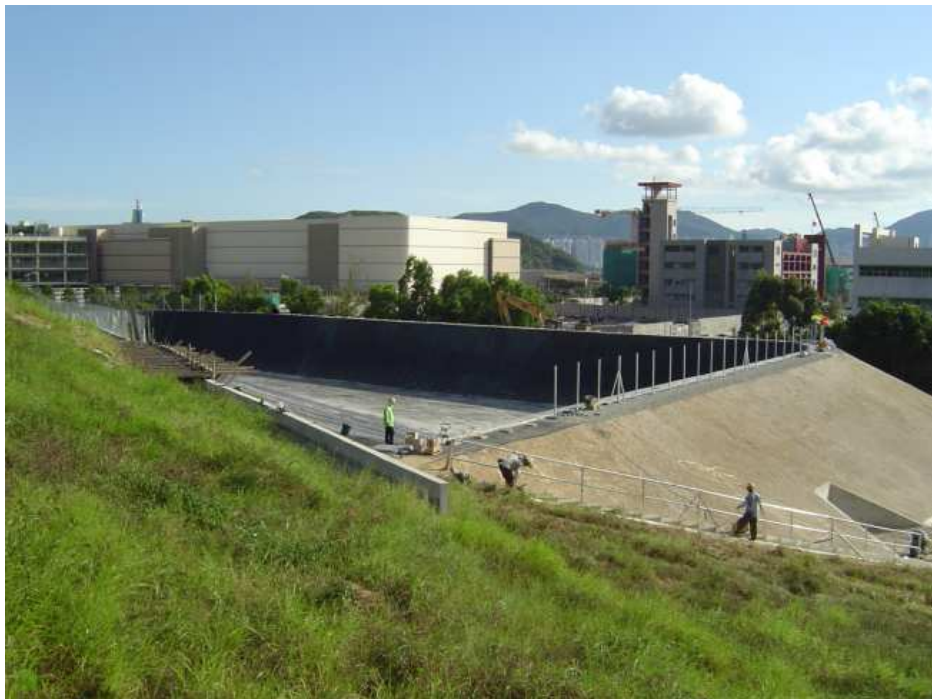
Reinforced embankment completed with HDPE lining
