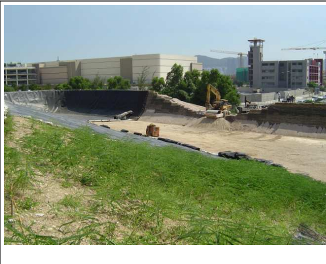
Construction of embankment
