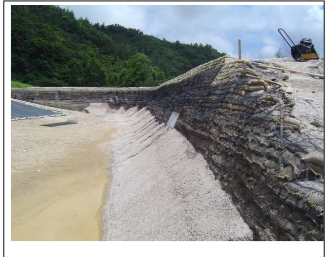
Wrap back TT045 geogrid at 70 degree slope
