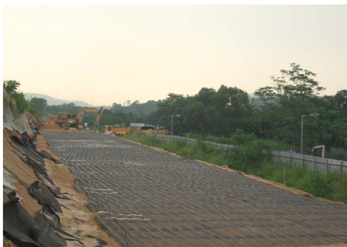
Figure 2 – Laying of Tenax TT090 geogrid (Slope SE5)
