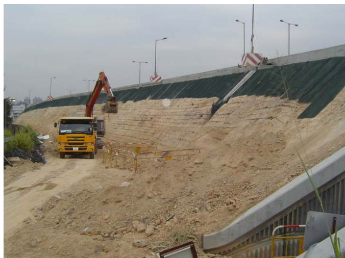
Figure 5 – Cutting back of slope facing
