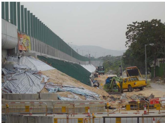
Figure 4 – Laying of erosion control mat
