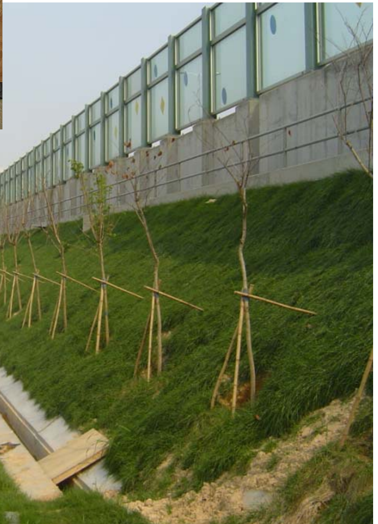
Figure 6 – During construction (Top) and after construction (Bottom) of reinforced fill slope
