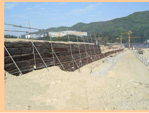
Building Up of Reinforced Fill Surcharge Embankment, Jan 2007
