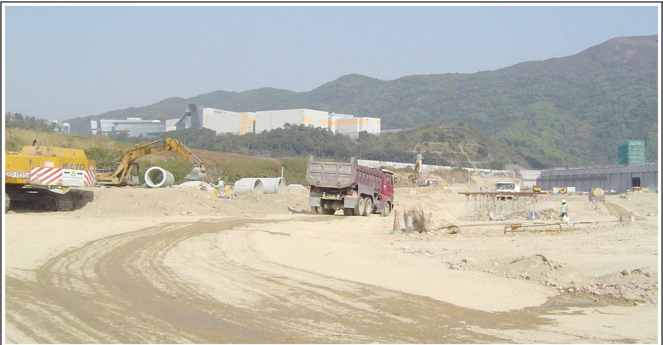
Removal of Surcharge Embankment after 9 months of Consolidation Jan 2008
