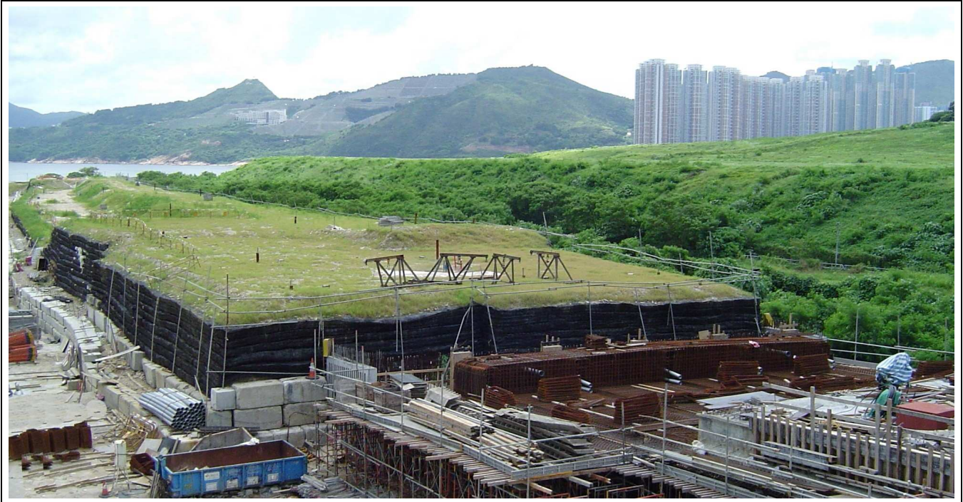
Overview of the Surcharge Embankment (300m x 50m x 8m), Jul 2007
