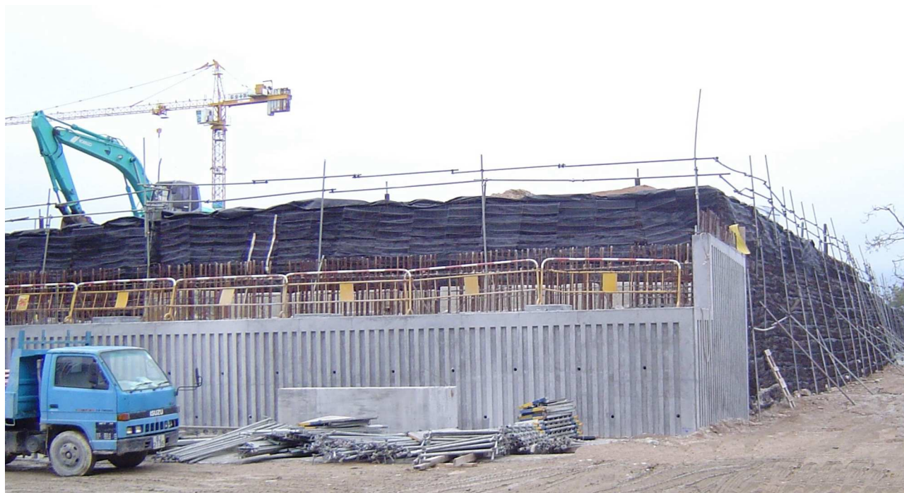
Completion of Surcharge Embankment, Mar 2007
