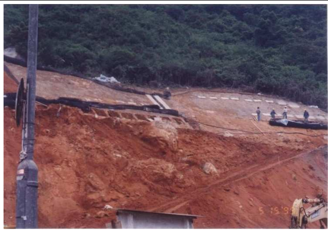
Site Preparation (May 1999)
