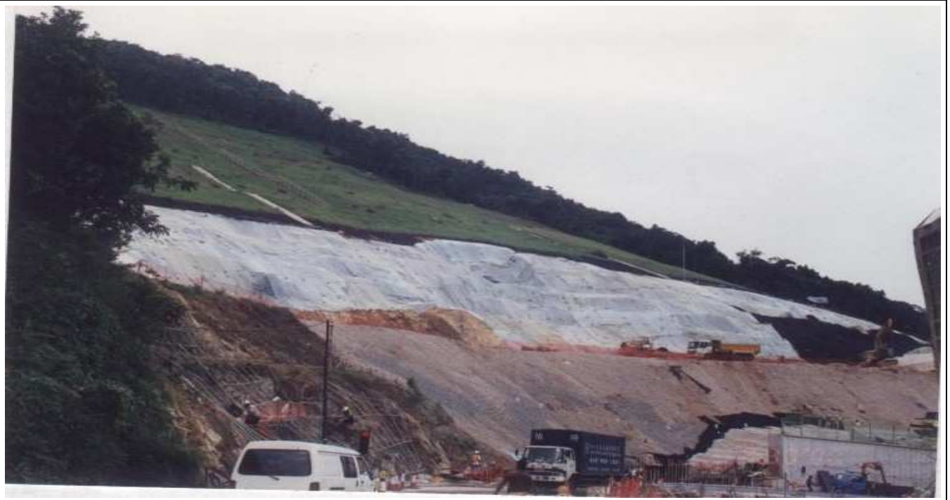
Construction Moved Toward the Toe (Aug 2000)
