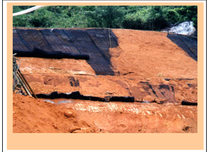
Installation of Multimatt (Nov 1999)
