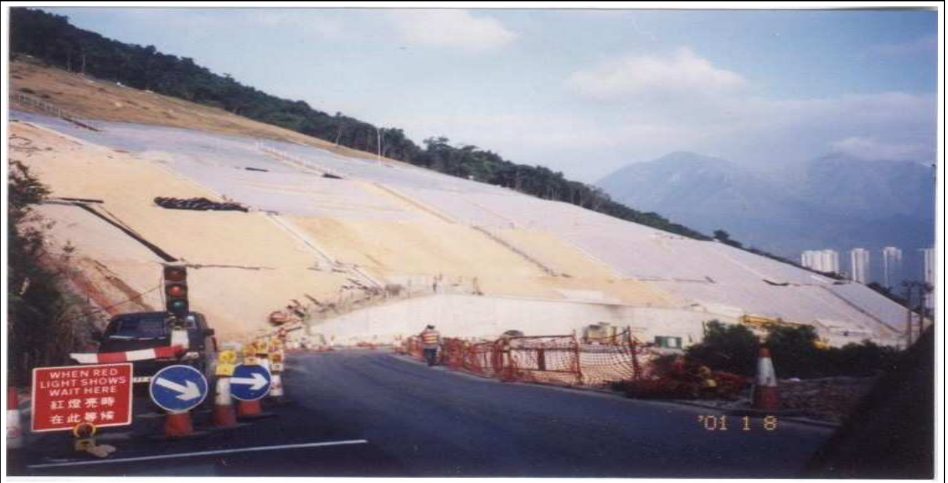
Hydroseeding Covered with Seed Protection New (Aug 2001)
