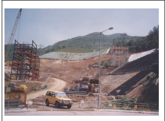
Above: Hydroseeding after installation (May 2000)
