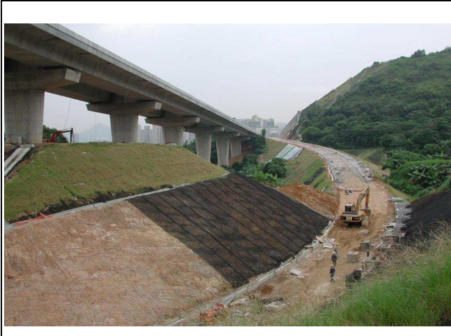
Above: Installation of TENAX Multimat 100
