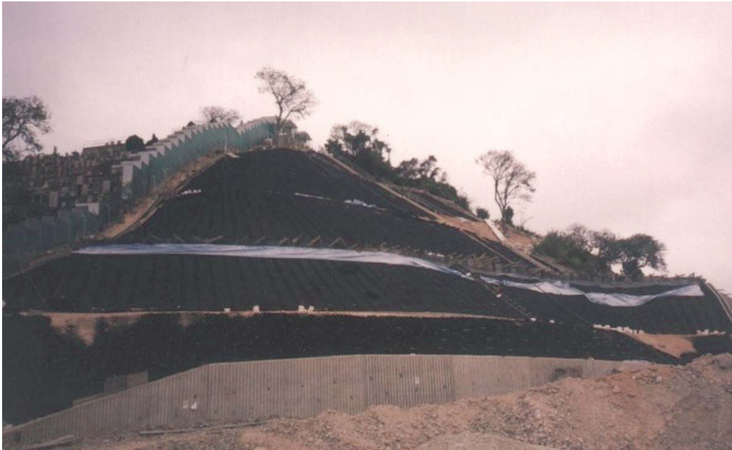
February 13, 2003 Laying of erosion control mat on soil infilled Miracell
