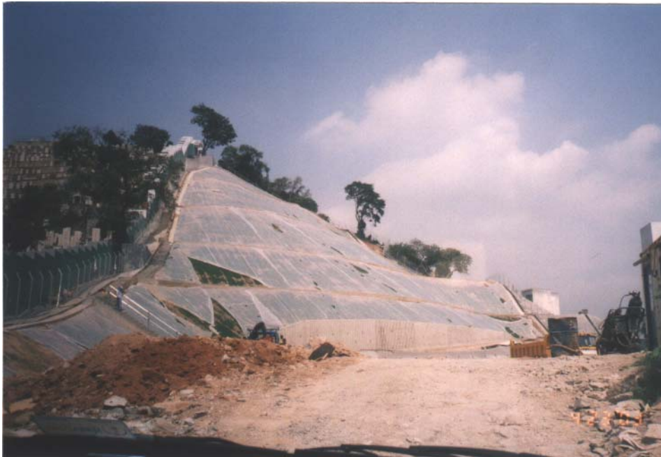
April 22, 2003 Application of hydroseeding and seed protection mat
