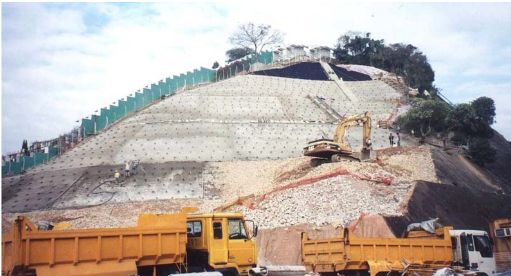
December 20, 2002 Laying of geotextile on shotcrete surface
