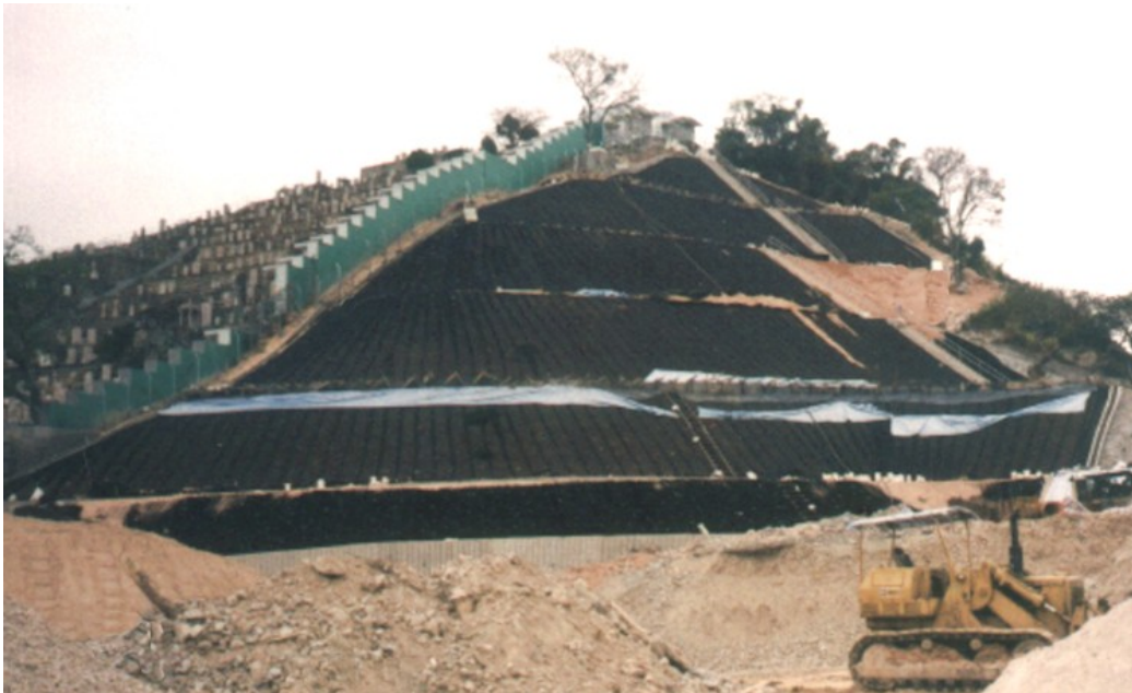
February 13, 2003 Spreading of soil into Miracell
