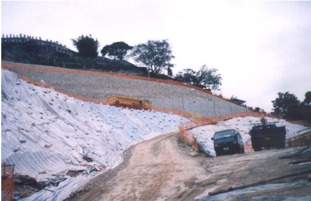
October 31, 2002 Rockfill slope ready for shotcrete
