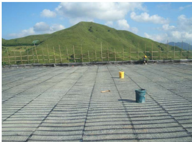
Photo 03 – Laying of Tenax TT Geogrid (3)
