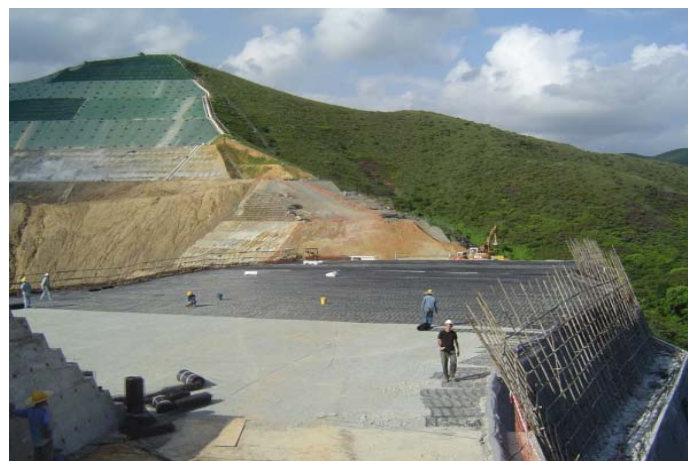
Photo 02 – Laying of Tenax TT Geogrid
