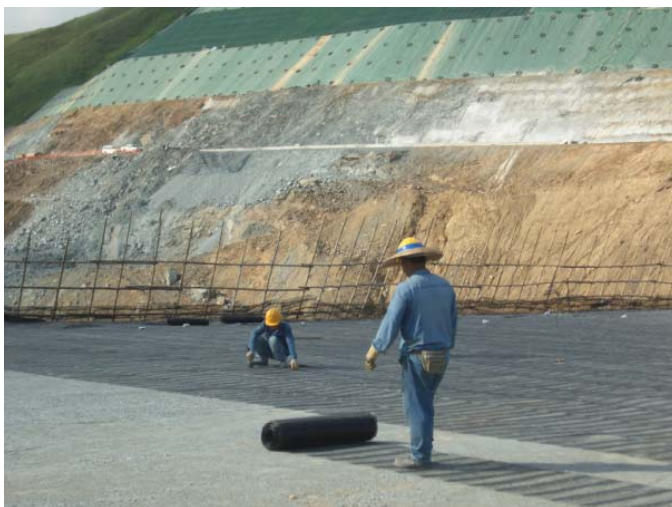
Photo 04 – Laying of Tenax TT Geogrid (4)
