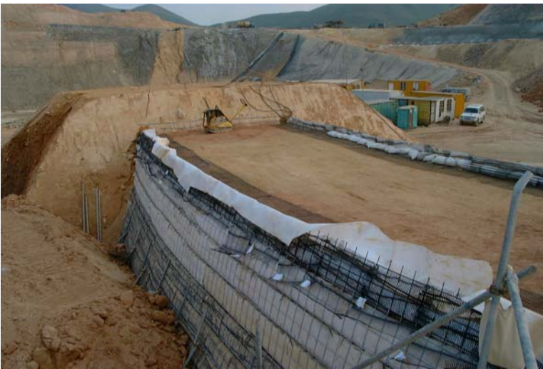
Photo 05 & 06 – Eastern Face of Reinforced Fill Embankment
