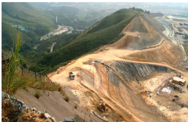
Photo 01 - Preparing the Slope
