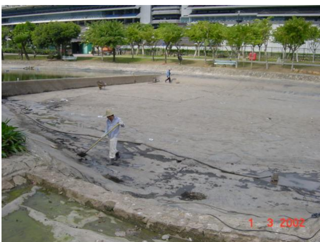
Desilting of Pond, July 2003. Minor Repair Works were Necessary After Bobcat Operation.
