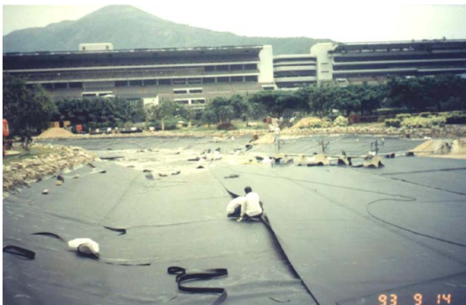
Laying Down of HDPE Membrane Waterproofing System at the Bottom of Pond, Sep 1993
