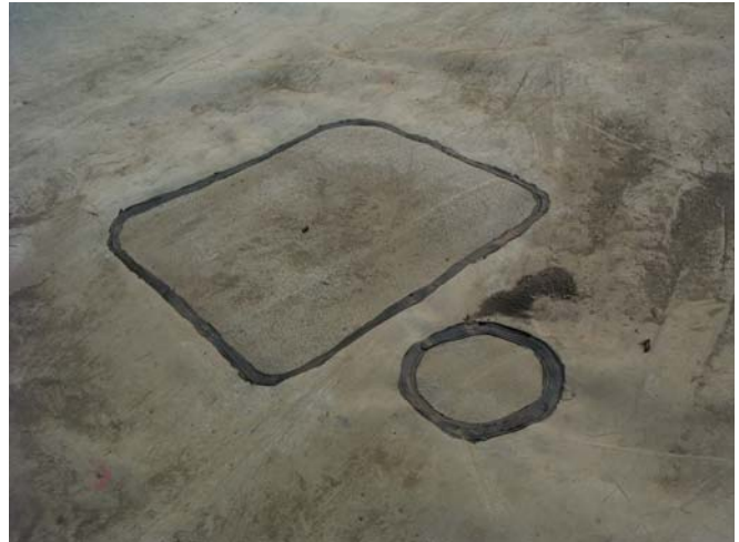
Repairing of HDPE Membrane, Sep 2005
