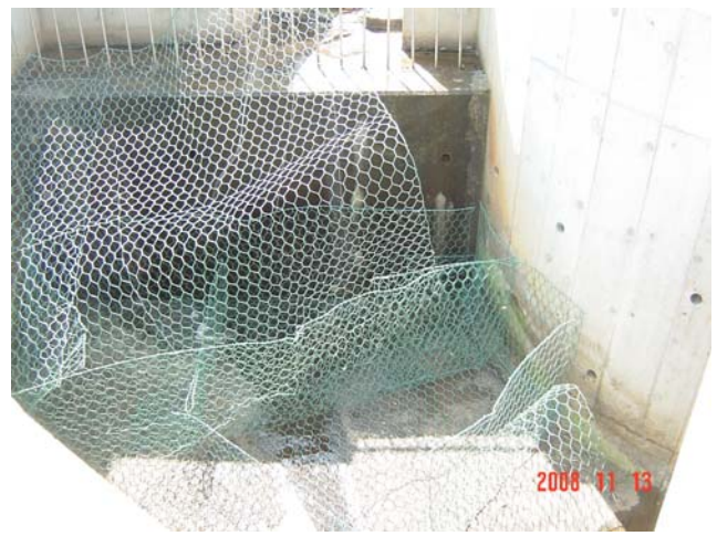
Laying Down of Gabion Unit
