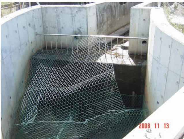
Laying Down of Gabion Unit
