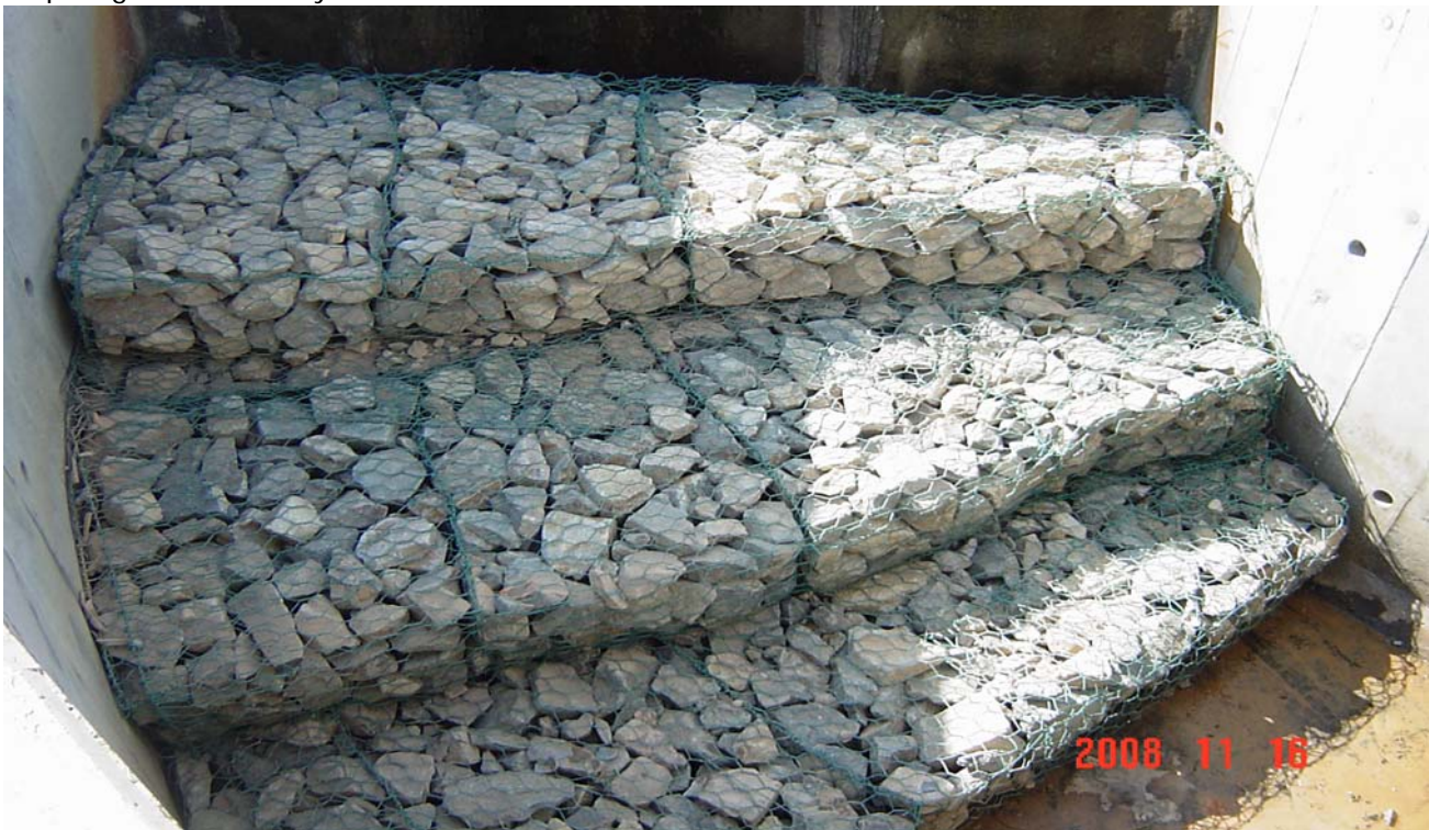
Trapezoidal Size Gabion Construction Along the Turn in Multi Layers
