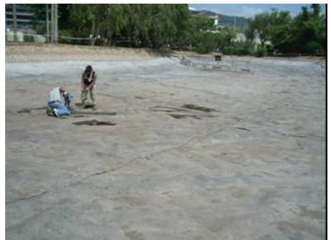
Repairing the Membrane, Sep 2005
