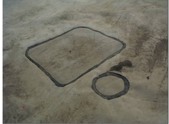
Repairing of HDPE Membrane, Sep 2005
