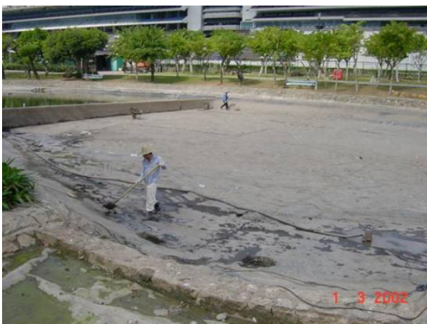
Desilting of Pond, July 2003
